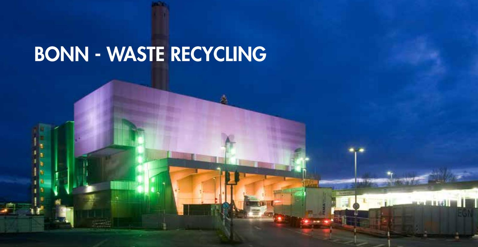
Recycling of the waste from Bonn and the surrounding region is carried out by Müllverwertungsanlage Bonn GmbH (MVA), a subsidiary of Stadtwerke Bonn (Bonn Public Utilities). Over 1,000 tonnes of waste, which has to be disposed of in a safe and environmentally friendly way, is delivered to it every working day. In a complex thermal process, the waste is first incinerated and then processed. Flue gases are created when the refuse is burnt.
