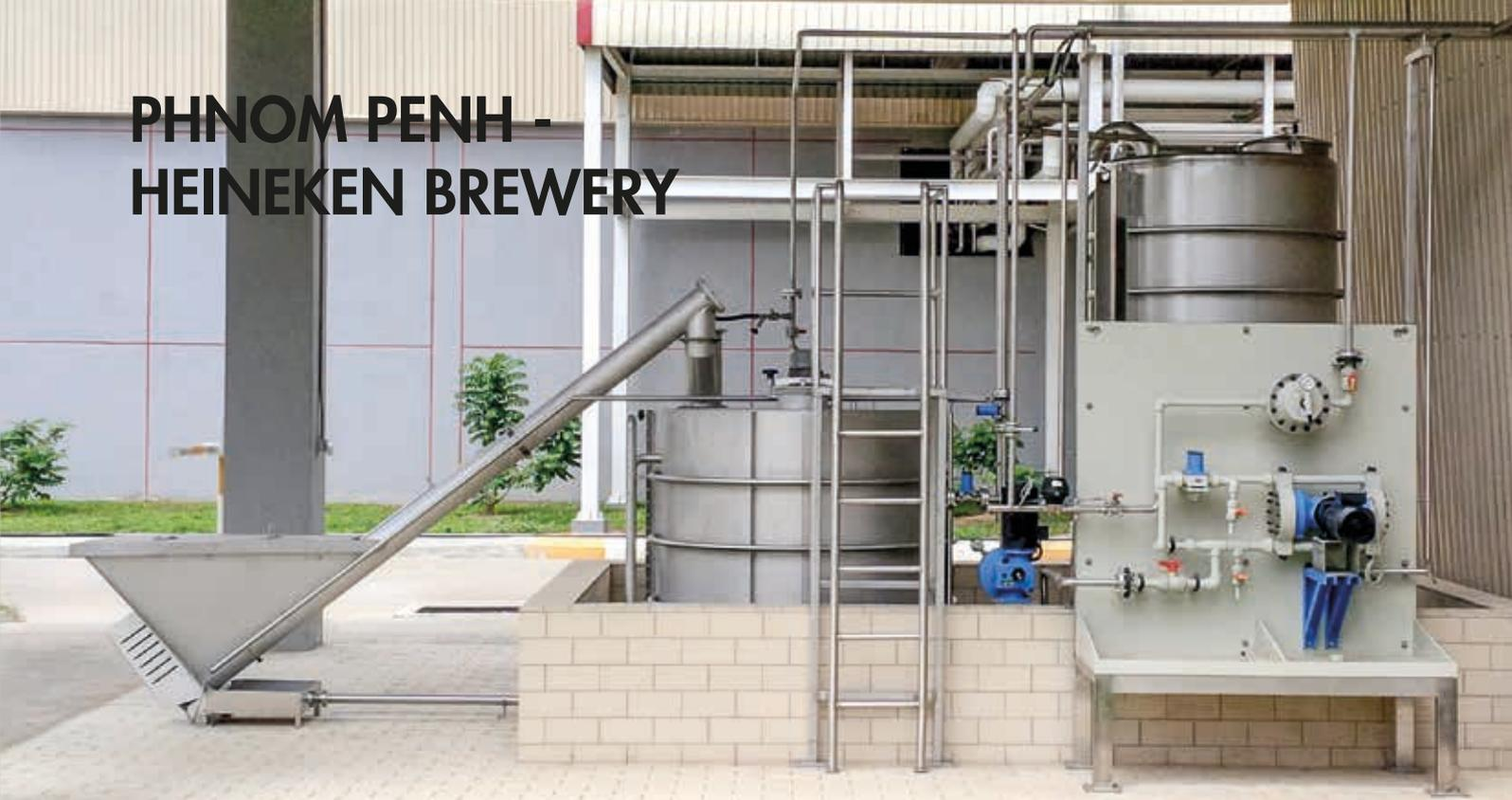
Approximately 50 million tons of caustic soda are produced annually and used in various ways in industry. **sera** has developed a cost-effective system solution specifically for use in the food industry, which has a variable but large demand for alkaline cleaning agents such as caustic soda. This enables safe and efficient preparation of caustic soda based on sodium hydroxide (NaOH) in solid form (pellets, flakes, pearls or powder) and water.
