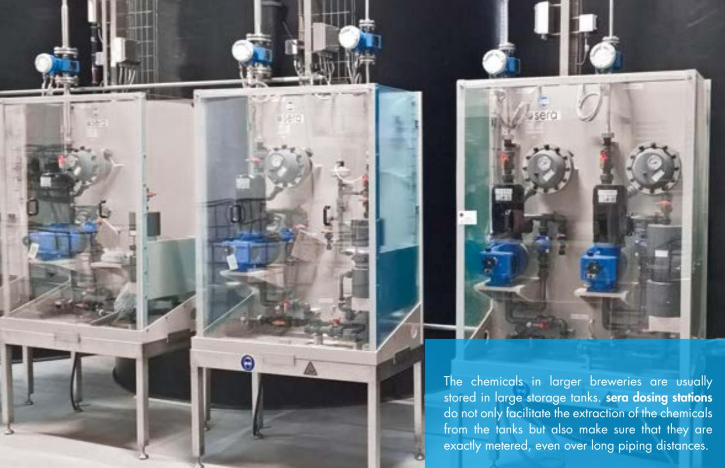
The chemicals in larger breweries are usually stored in large storage tanks. **sera dosing stations** do not only facilitate the extraction of the chemicals from the tanks but also make sure that they are exactly metered, even over long piping distances.
