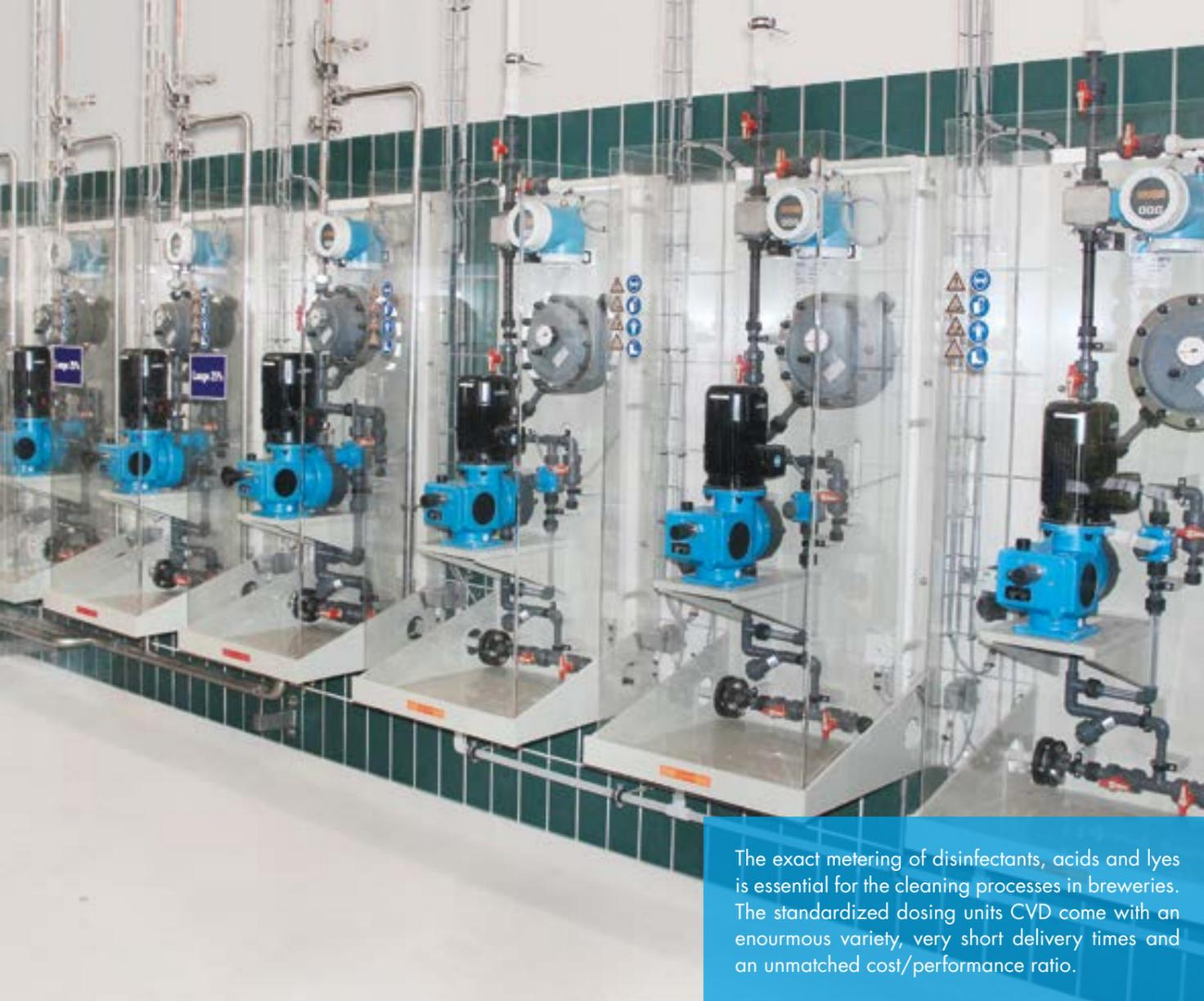
The exact metering of disinfectants, acids and lyes is essential for the cleaning processes in breweries. The standardized dosing units CVD come with an enormous variety, very short delivery times and an unmatched cost/performance ratio.
